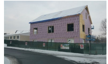
Upper school building addition in progress
