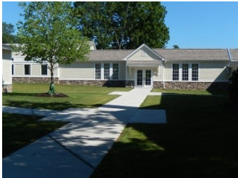
Lower School New Addition
