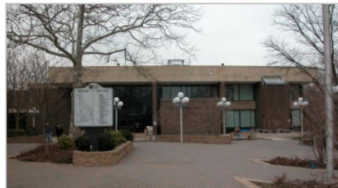
Existing Library before 3 rd floor addition
